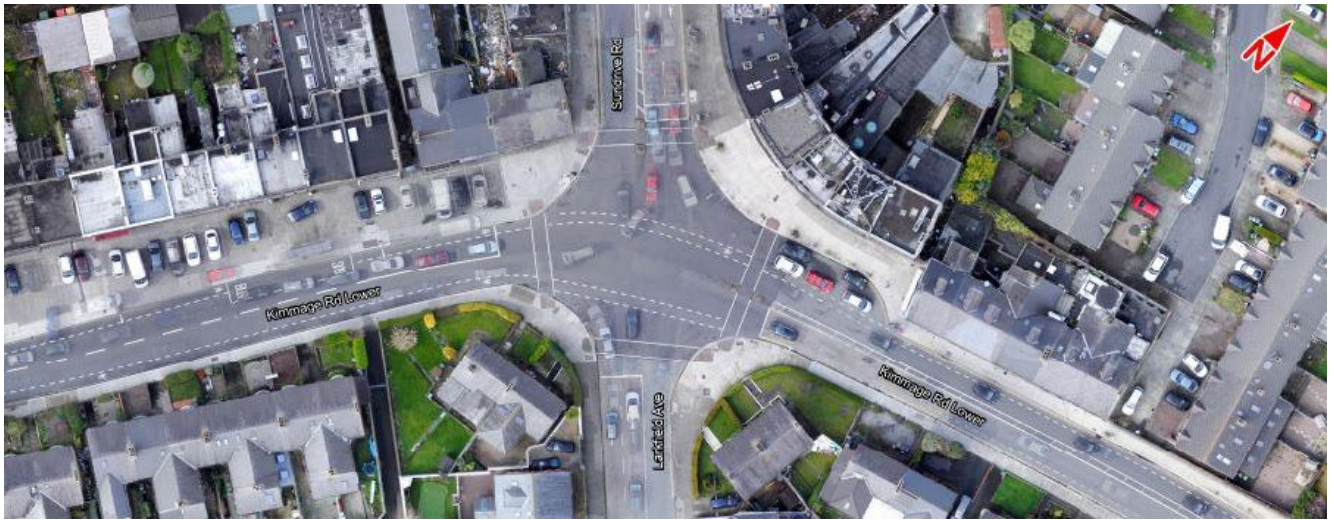
Image 6.3: R817 Kimmage Road Lower / Sundrive Road and Larkfield Avenue Four-Arm Signalised Junction
